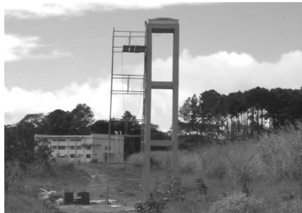
Fig. 1. RCS support pylon. The pylon can be seen in the foreground. This picture was taken while the electrical wiring of the turntable was being installed. The height of the pylon is 7.95 m and its width is 1.4 m.
